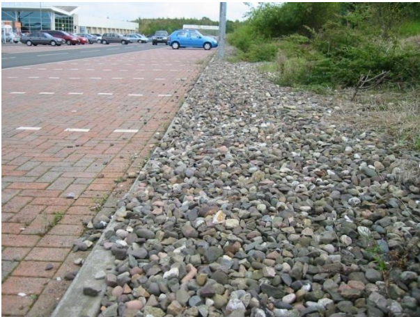
Figure 4a: Permeable paving
