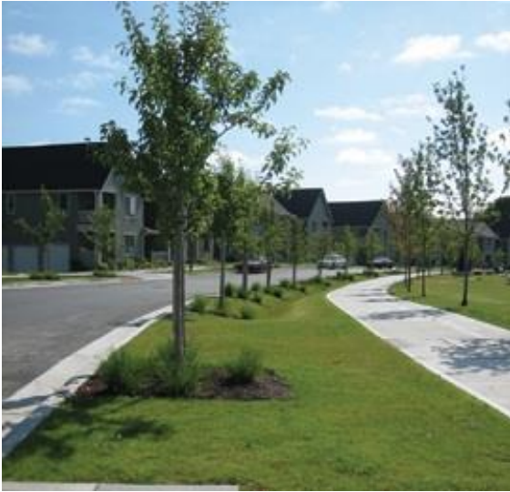
Figure 4c: Swale along road corridor
